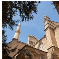
02 Gothic buttresses and minaret
