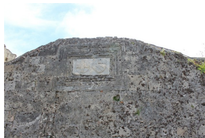
02 The two coats of arms above
