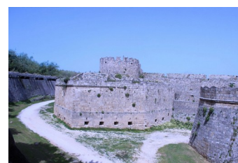
06 Bastion and Terreplein of Spain
