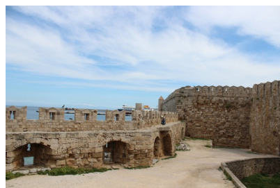
05 The sea wall and the harbour
