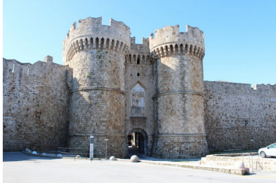
01 The gate and its two towers
