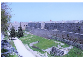
05 The moat beside the curtain wall
