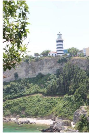
Fig. 6: Sile Light House, Sile, Turkey Source: the MIS/ETC/2619 ALECTOR Project Record
